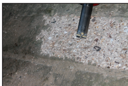
ROUGHENING CONCRETE
