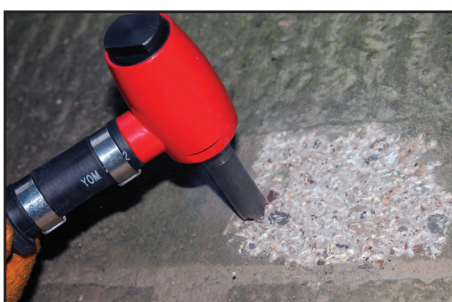
REDUCING LEVELS ON CONCRETE
